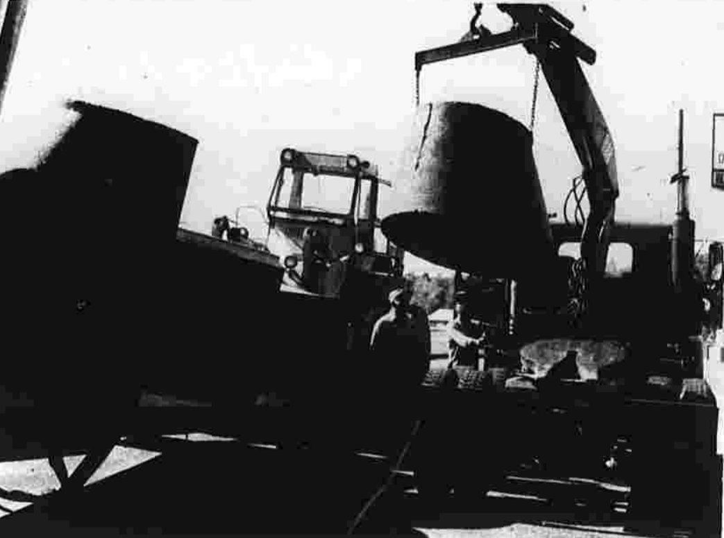
Workers unload one of the huge concrete pipes from a trailer with a 72,000-pound load which sank into the pavement at Manchester Motor Sales. (Herald photo by Chastain)
